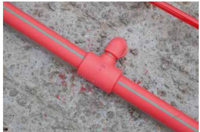
Assembly precast concrete ceiling
