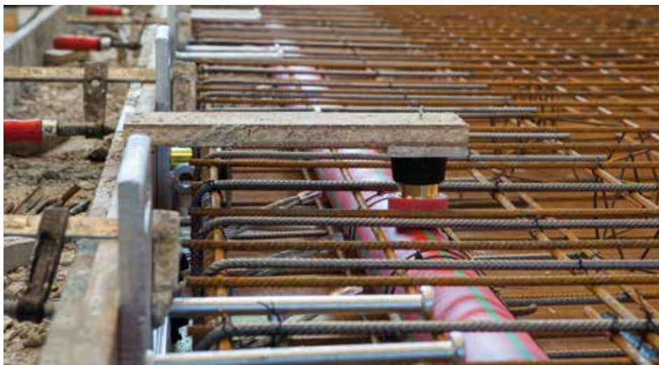
Prefabrication concrete wall
