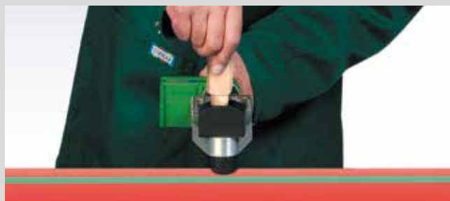
Heat-up of pipe...
